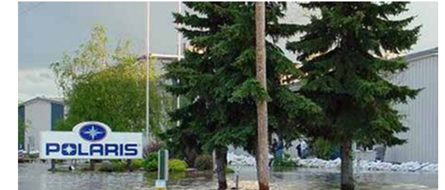
The Polaris plant as the flood waters were rising in 2002.
