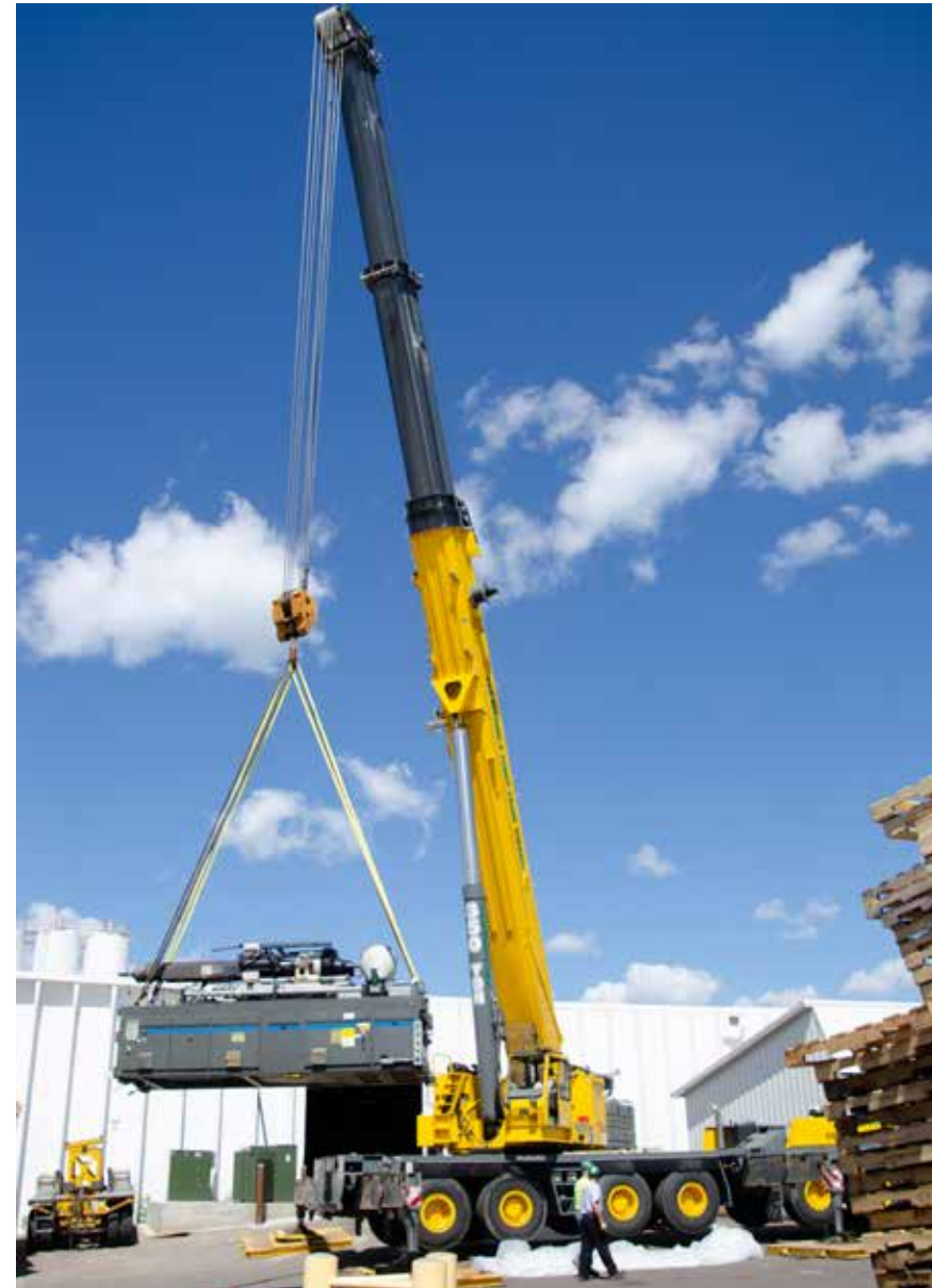
Moving in one of three sections of a new 1,500-ton press.
