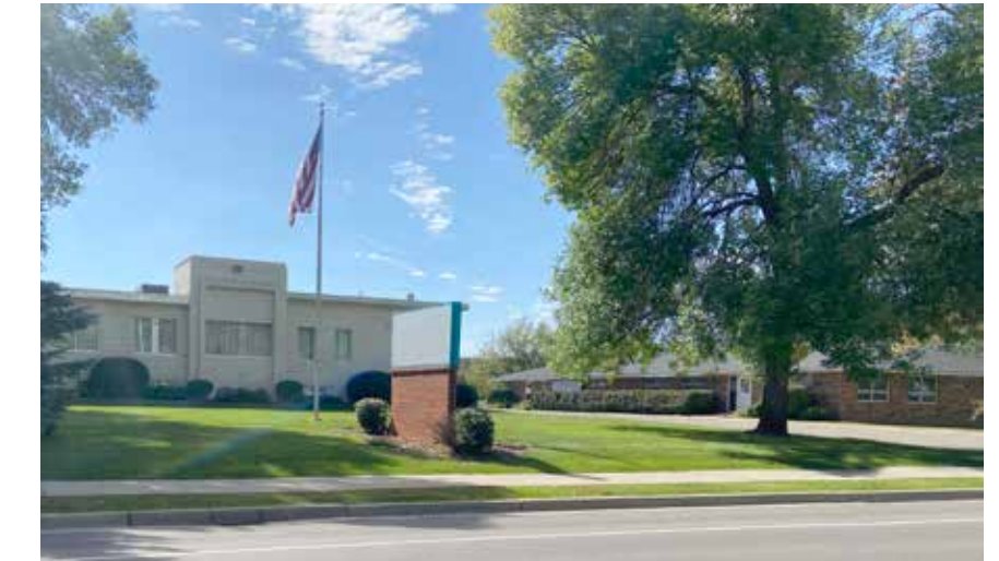
The former Rush City Hospital and Clinic, in the process of renovation to house Plastech production employees who are documented immigrant workers.
