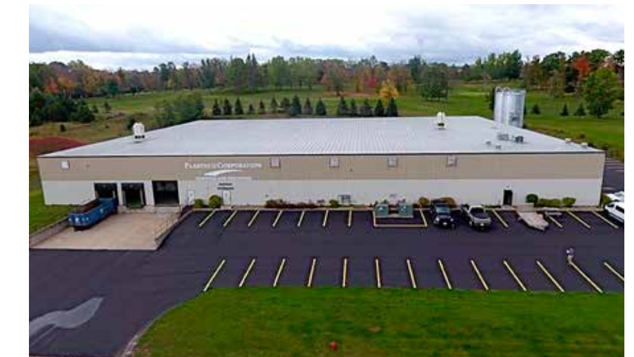
Aerial view of the Frederic plant.
