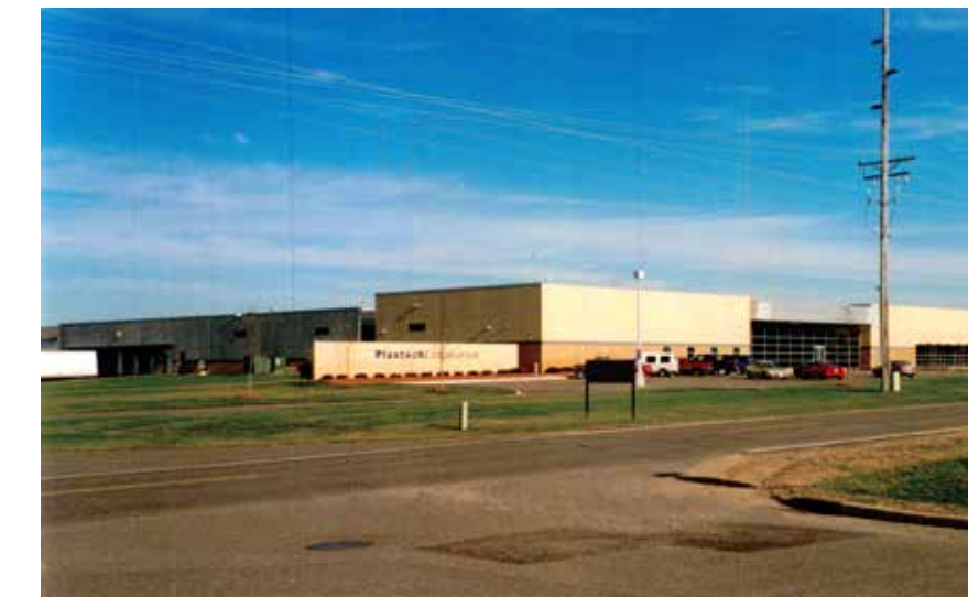
Plastech's Amery complex, 2002.
