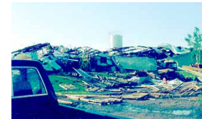
The North States Industries plant after the Siren tornado, 2001.
