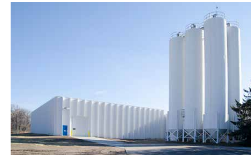
Exterior of the new addition, November 2012.
